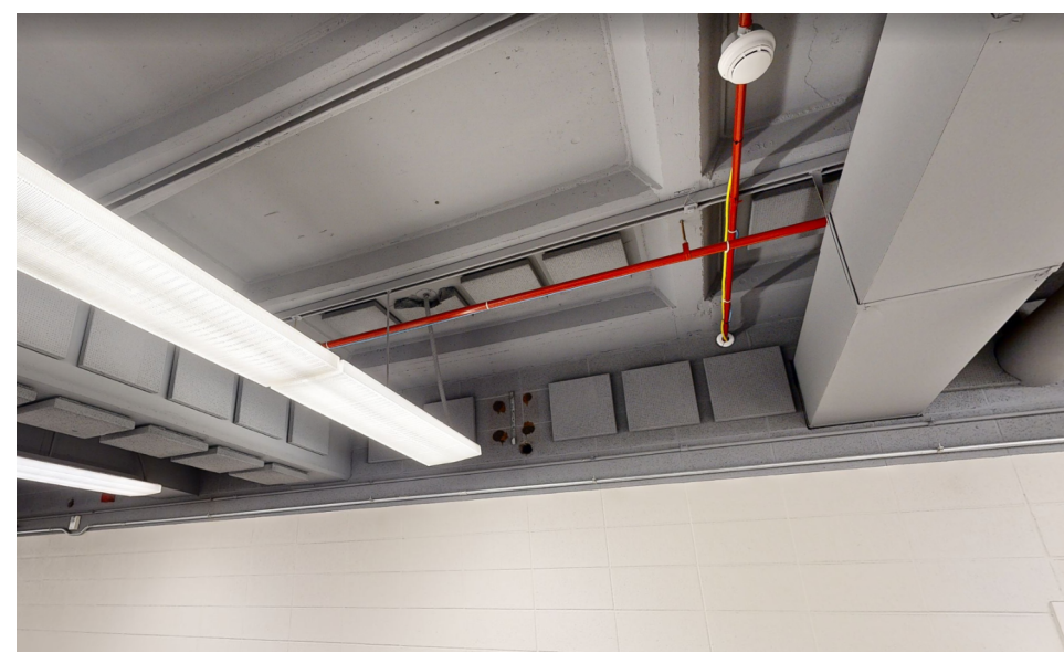
IMAGE 1 - EXAMPLE OF EXISTING ACOUSTIC PANELS AND ADHESIVE
